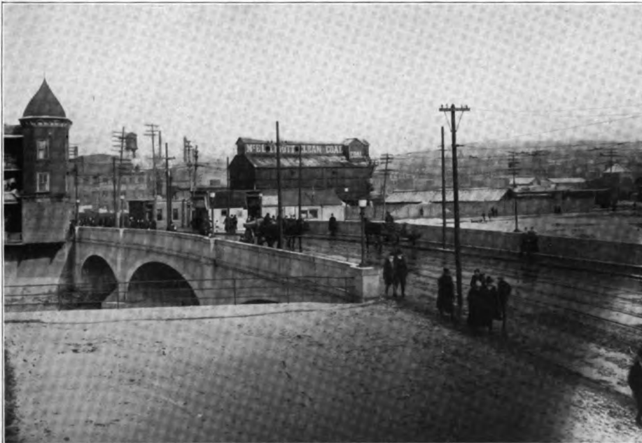
THE BROOKLYN BRIDGE, CARRYING BANK STREET OVER THE NAUGATUCK RIVER
