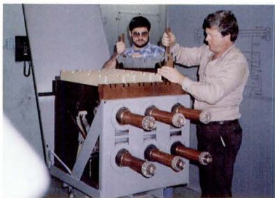
Technicians Repair Electronic Equipment.
