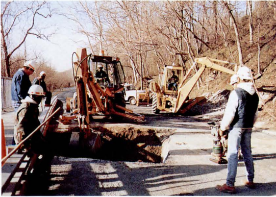
Excavation to Locate Pipeline
