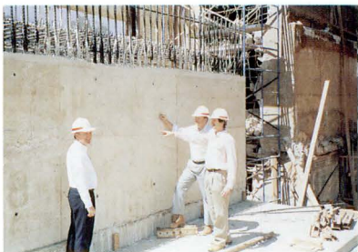
Engineers in Field Inspection.
