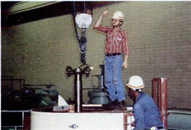
Routine Pump Maintenance. Digitized by Google
