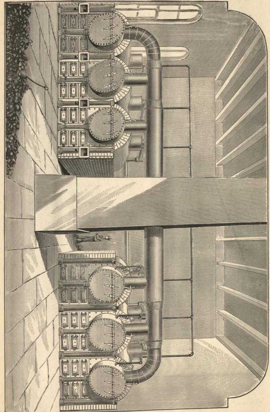
PLATE II.—Sectional View of Inside of Boiler House.
