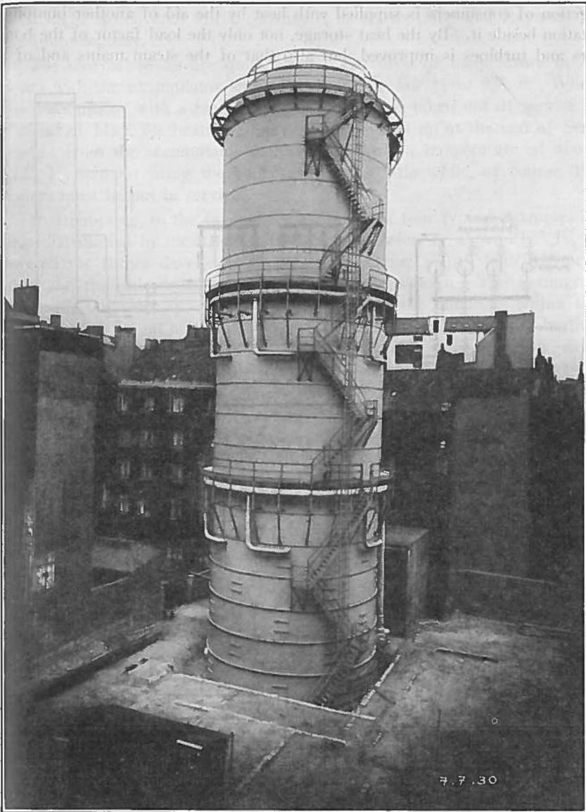
FIG. 3—Large Capacity Hot Water Accumulator
