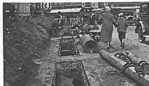
Installing ADSCO Casing in Wilkes-Barre, Pa.
