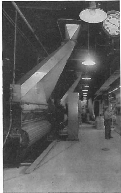
This view inside the nearly completed plant shows a control panel (at right), chain grates (left) and a chute (above) from a coal bunker.
