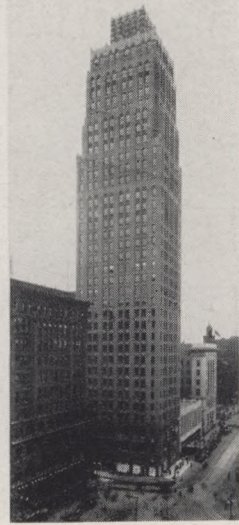
DAVID STOTT BUILDING
