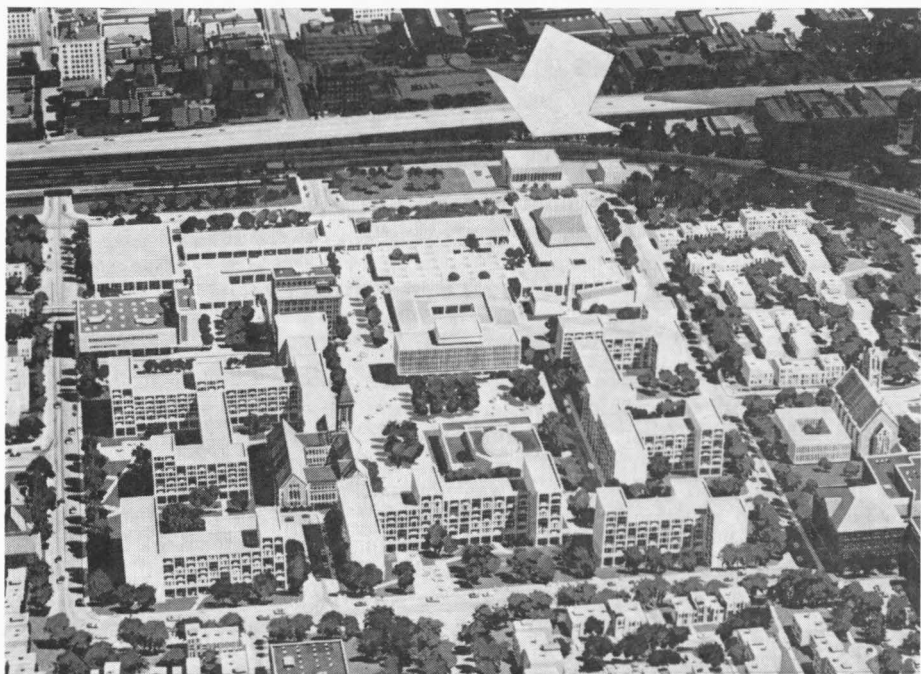
FIG. 1—Allegheny Center's facilities—stores, offices and living quarters—have a pleasant climate in common through central heating-cooling plant (arrow).
