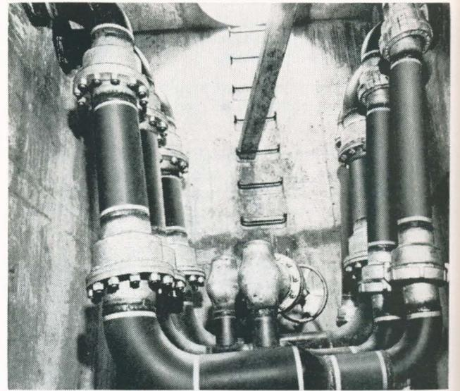
FIG. 3 — Ball joint installation in the high-temperature water system manholes.
