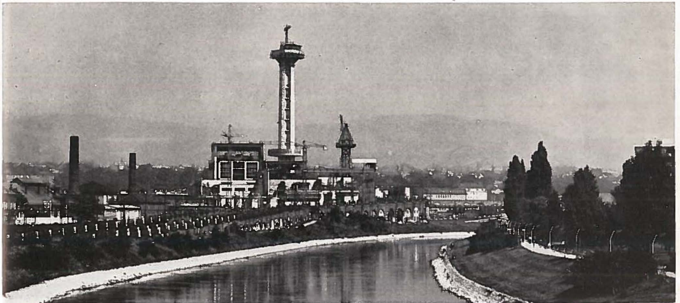
SPITTELAU INCINERATION-STEAM PRODUCING PLANT—Vienna, Austria . . . . . Page 12
