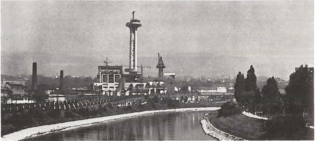
General view of the Spittelau garbage incinerating and steam producing plant which provides district heating for the city of Vienna on an economical basis as well as feeding electricity into the Austrian grid.
