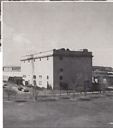
Arlington Heating Plant Arlington, Virginia
