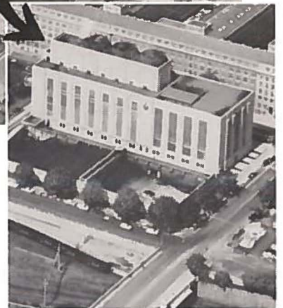
Central Heating Plant Washington, D. C.
