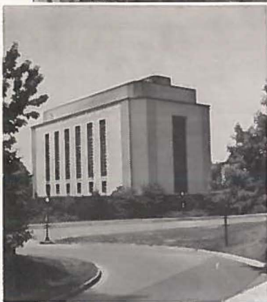
West Heating Plant Washington, D. C.
