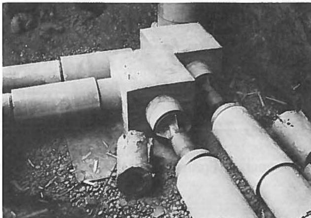
Fig. 9 — Factory-made angle fixed point element.
