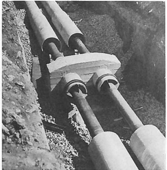
Fig. 10 — Factory-made straight fixed point element.
