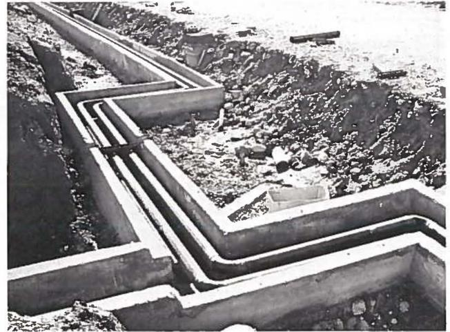
Fig. 4—Expansion in the buried network is taken up by simple U off-sets.
