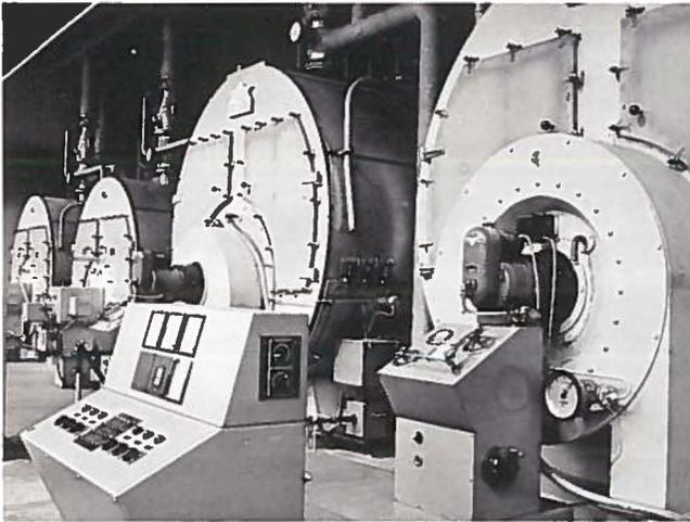
Fig. 3—Rotary cup burners atomise heavy oil in this district heating station.
