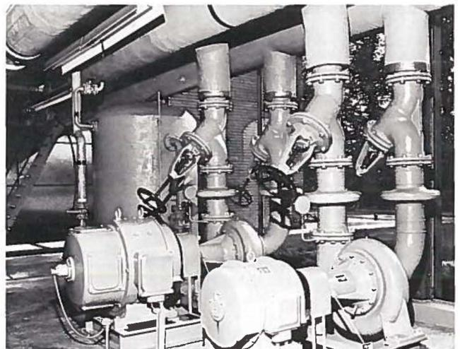
Fig. 2—Variable speed pumps save power with off-peak network loads.
