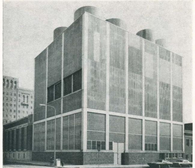
Fig. 1 — View of the Franklin Station. Taller portion in foreground is refrigeration section and cooling towers. Lower portion in background is electric generation area.
