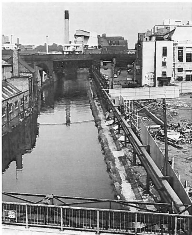
Fig. 5—Looking east along Nottingham Canal towards London Road, the high pressure hot water mains can be seen on the right bank and in the foreground.
