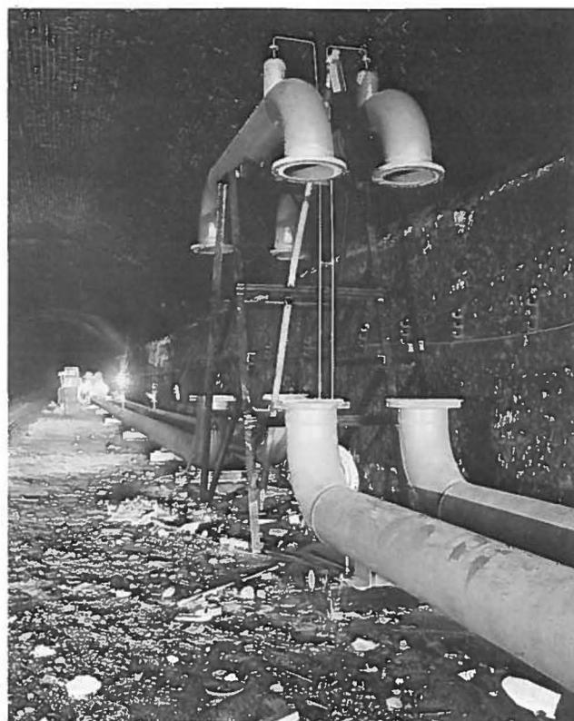
Fig. 6—Heating tunnels being installed within the old railway tunnel leading to Victoria Centre.
