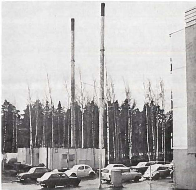
Fig. 4—Transportable boiler plant, Finland, gives local heat supply for initial stages of district heating, pending build-up of load large enough for using power station waste heat when a number of such schemes are connected together.
