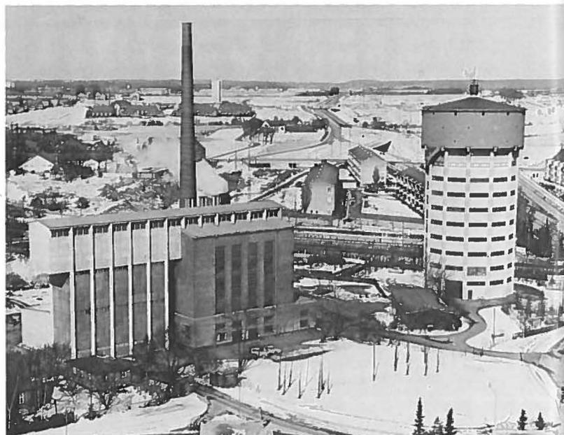
Volud refuse incineration plant used in conjunction with an ITOC turbine to supply a Danish heating network.
