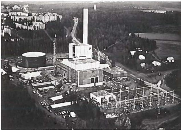
Fig. 5—Martinlaakso CHP station, Vantaa: electric output 60 MW; district heat output 117 MW.
