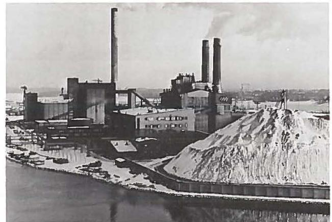
Fig. 4—Hanasaari CHP stations, Helsinki. Hanasaari B, left, two back-pressure units: electric output 2 x 113 MW; district heat output 2 x 203 MW (+ 56 MW auxiliary boiler). Hanasaari A, right, two extraction-condensing units: electric output 182 MW maximum (79 MW back-pressure); district heat output 193 MW.
