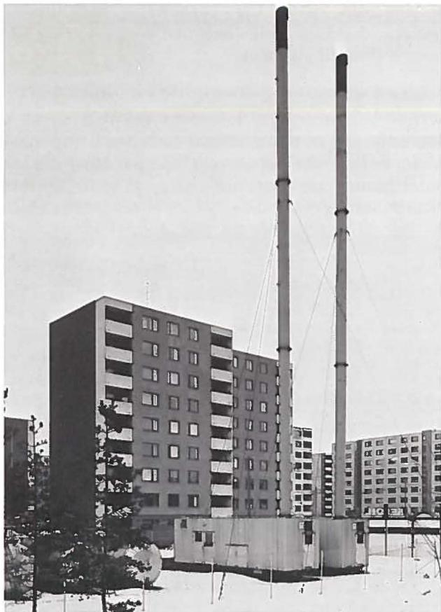
Fig. 6—Two typical transportable heating plants in operation on a newly built area: heat output 2 x 4 MW.
