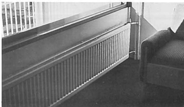
Fig. 6—Typical parallel plate room heater.
