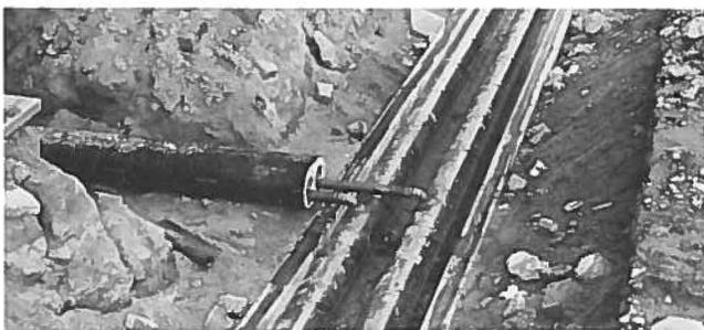
Fig. 4—Customer service tap of pipelines, Turku.
