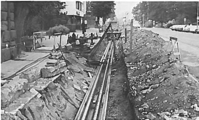
Fig. 3—New district heating pipeline, Turku. Note customer tap at center.
