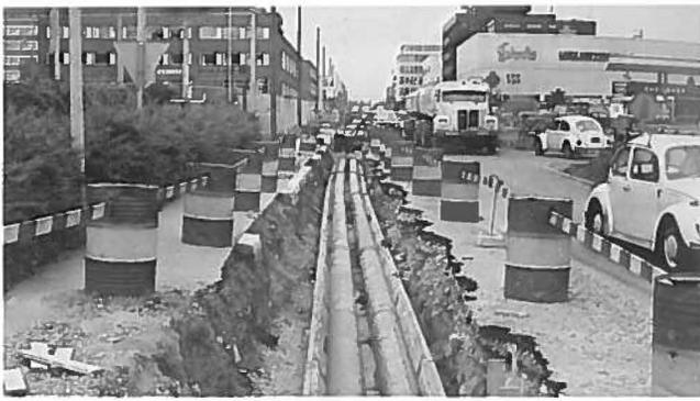
Fig. 1—District heating pipeline extension, Helsinki.
