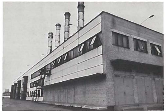
Fig. 3—Moscow: central heating plant serving housing project.
