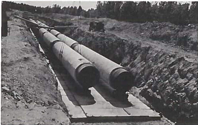
Fig. 7—Leningrad: prefabricated concrete tunnel panels, five sections.
