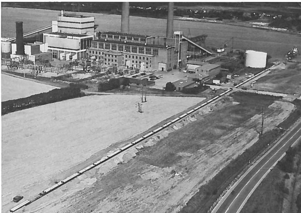
Combined heat and power station on the island of Masnedo, Denmark, showing the sea-crossing section of heat mains being prefabricated and assembled prior to installation under the sea.
