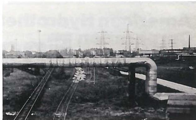
Moscow District Heating System — 1400 MM hot water supply and return lines in vicinity of combined heat and power plant.
