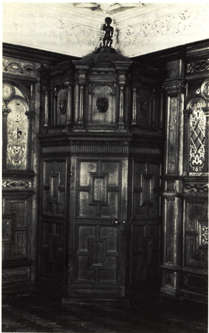
Figure 1. Draught-proofing inner porch from Sizergh Castle, Westmorland, 1382.
