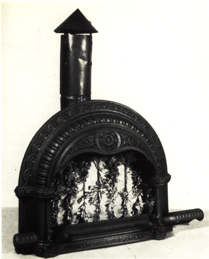
Figure 21. Gas fire with tufted asbestos radiants, 1882.
