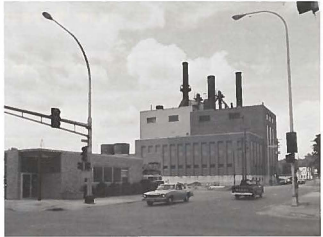
A new building was erected adjacent to the existing municipal power plant to house the heat exchangers to convert the steam to hot water for the new system.
