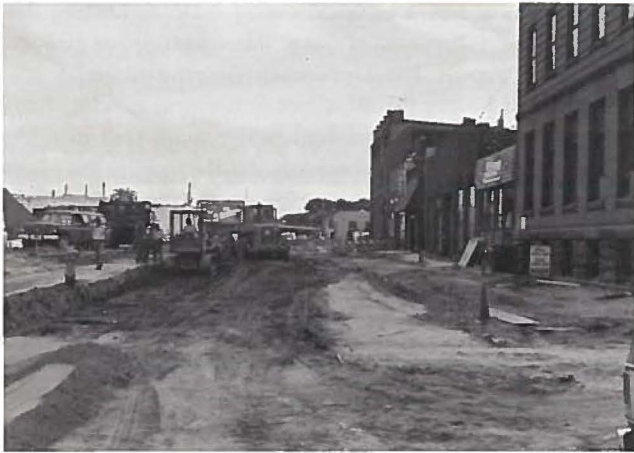
The streets of Willmar have been torn up for total redevelopment.
