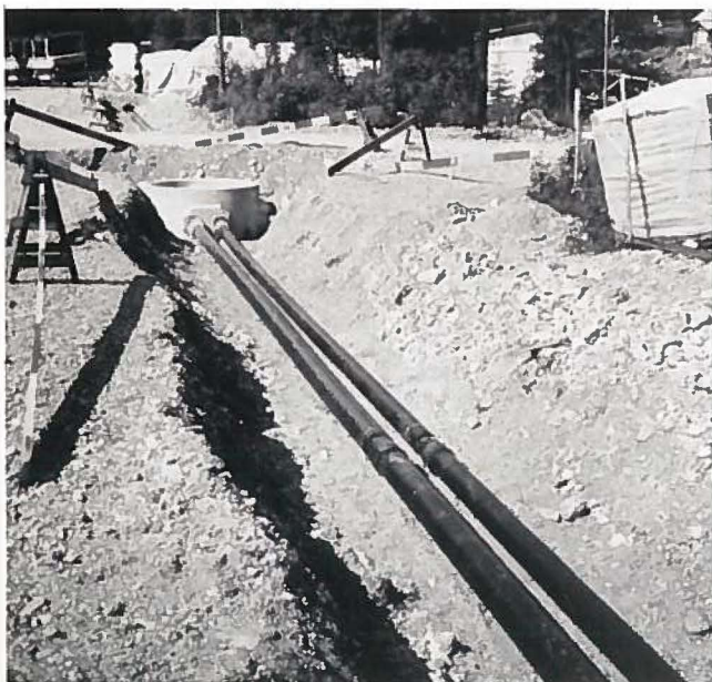
Figure 2 DH Construction Site in Kouvola
