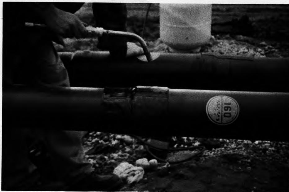
*The ends of the joint sleeve were sealed with a heat-shrink material to keep groundwater from entering the insulation.*
