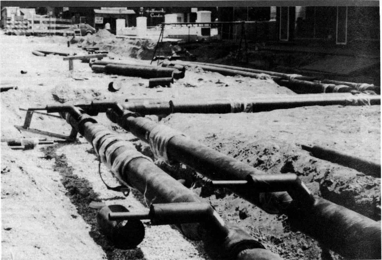
*Installation of district heating system in Willmar. Following page: Willmar's district heating plant and downtown after completed pipe installation.*
