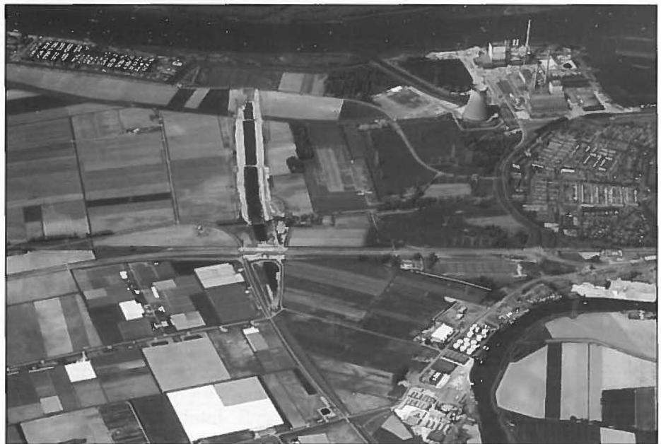
This is an aerial view of the glass greenhouses of Plukmadese Polder with the heat-delivering Amer Power Station in the upper right.
