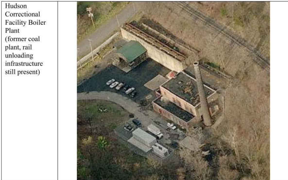
Figure 2: Hudson Correctional Facility Boiler Plant
