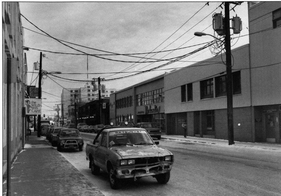
Downtown Fairbanks prior to the utilidor construction.
