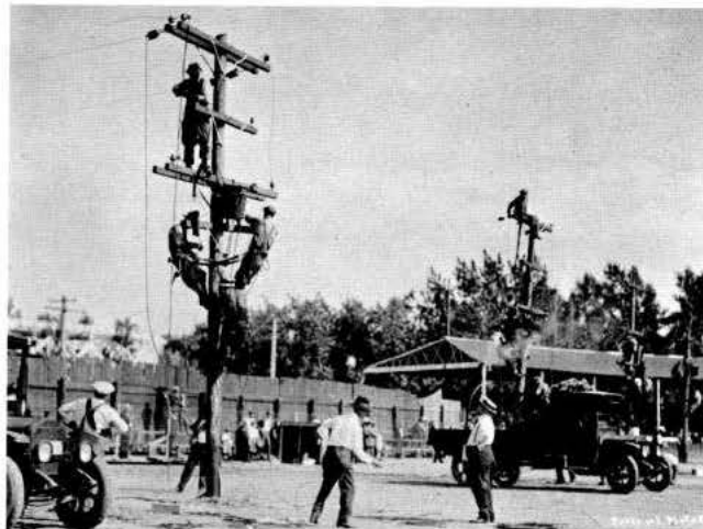
Linemen of the Denver Gas & Electric Light Co. install transformers on distribution line power poles using up-to-date equipment, including a modern line truck of the Twenties. This was an intracompany competition at the annual picnic in Denver.
