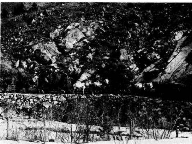
A ten-horse team pulls a section of generating unit five miles up rugged Boulder Canyon during construction of Boulder Hydroelectric Plant, which went into operation in 1910. The horses to the rear are relief teams.
