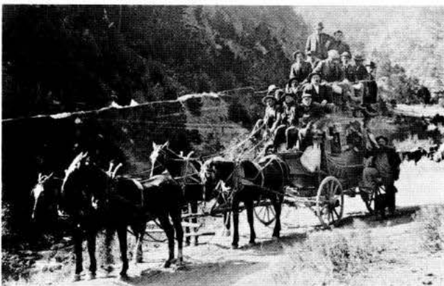
Workers being taken to construction site of Barker Dam near Nederland in the first decade of this century.
