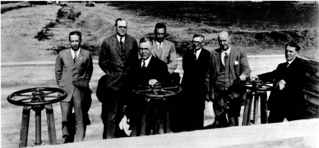
Natural gas was introduced in Denver on June 23, 1928, through pipeline constructed by Colorado Interstate Gas Co. from Texas Panhandle gas fields. This photo shows ceremony turning gas into the city mains of Denver. Denver Mayor Ben F. Stapleton is third from left, Guy W. Faller, PSCo vice president, is third from right.
