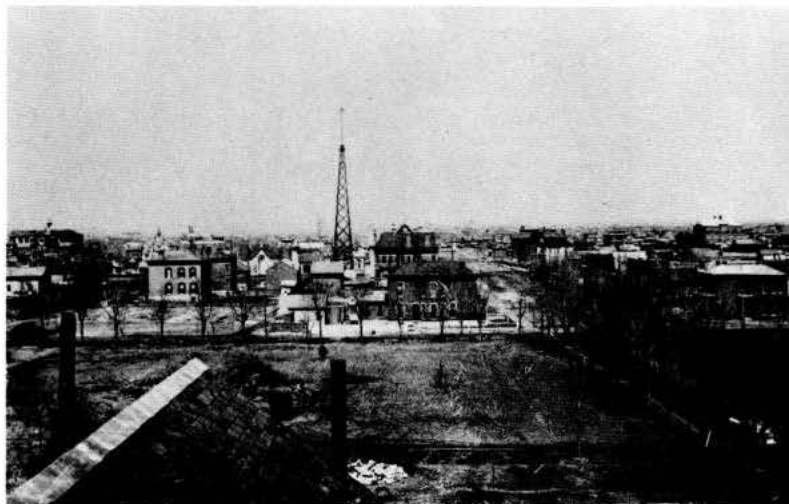
Lighthouse of the Plains is what such a street lighting tower was called in the early 1880's. There were eight in Denver, 150 to 200 feet high, each supporting eight 3,000-candlepower arc lights. This one was on Capitol Hill.
