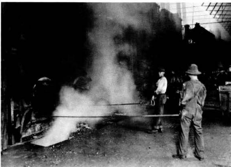
Removing the coke from the huge retorts in this early day gas manufacturing plant was hot, tedious, dangerous work. Coke was all that remained of coal baked to release gases used to illuminate Denver's first street lights in 1870. Such gas was later used for illuminating homes and businesses and for cooking. There was only one manufactured-gas house heating customer in January 1922, and the number grew to 730 by 1928, when natural gas arrived from Texas.
