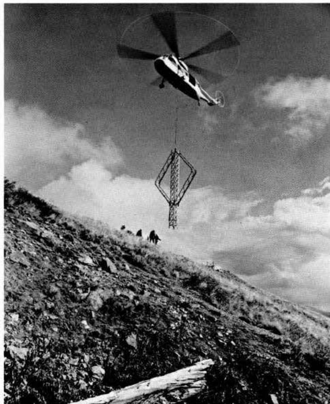
Helicopter replaces the horse in transmission line construction in the mountains.
