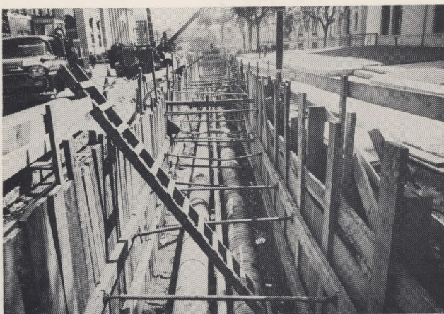
Fig. 2—Prospect Street Pipe-Line Excavation Looking South from Atheneum North—June 23, 1961.
