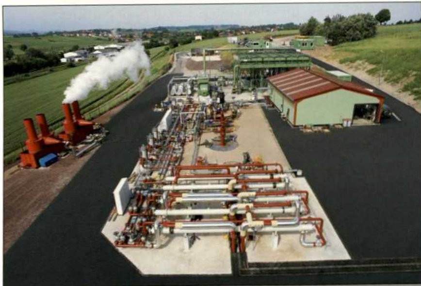
The Soultz geothermal power plant. At the back of the project site is the Organic Rankine Cycle power unit; in the middle of the site are the three geothermal wells; at the front is the cooled geothermal loop. The town of Soultz-sous-Forêts is in the background, about a kilometer away. CAPTION COURTESY OF A. GENTER; PHOTO COURTESY OF GEIE.
