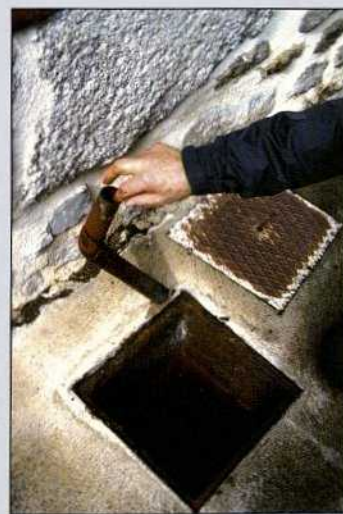
Diagram of the hot waters from le Par spring flowing down the street (upper right corner of the photo), entering a house, and passing beneath the floor. The large basin retains heat. REPRINTED COURTESY OF GÉOTHERMIA, MUSÉE EUROPÉEN DE LA GÉOTHERMIE ET DU THERMALISME.
