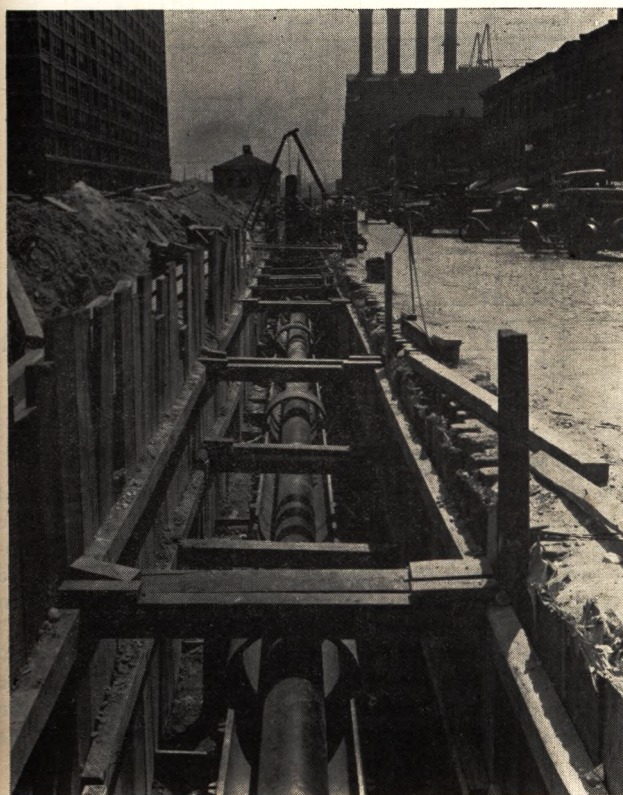
Cast Iron Conduit under Construction
