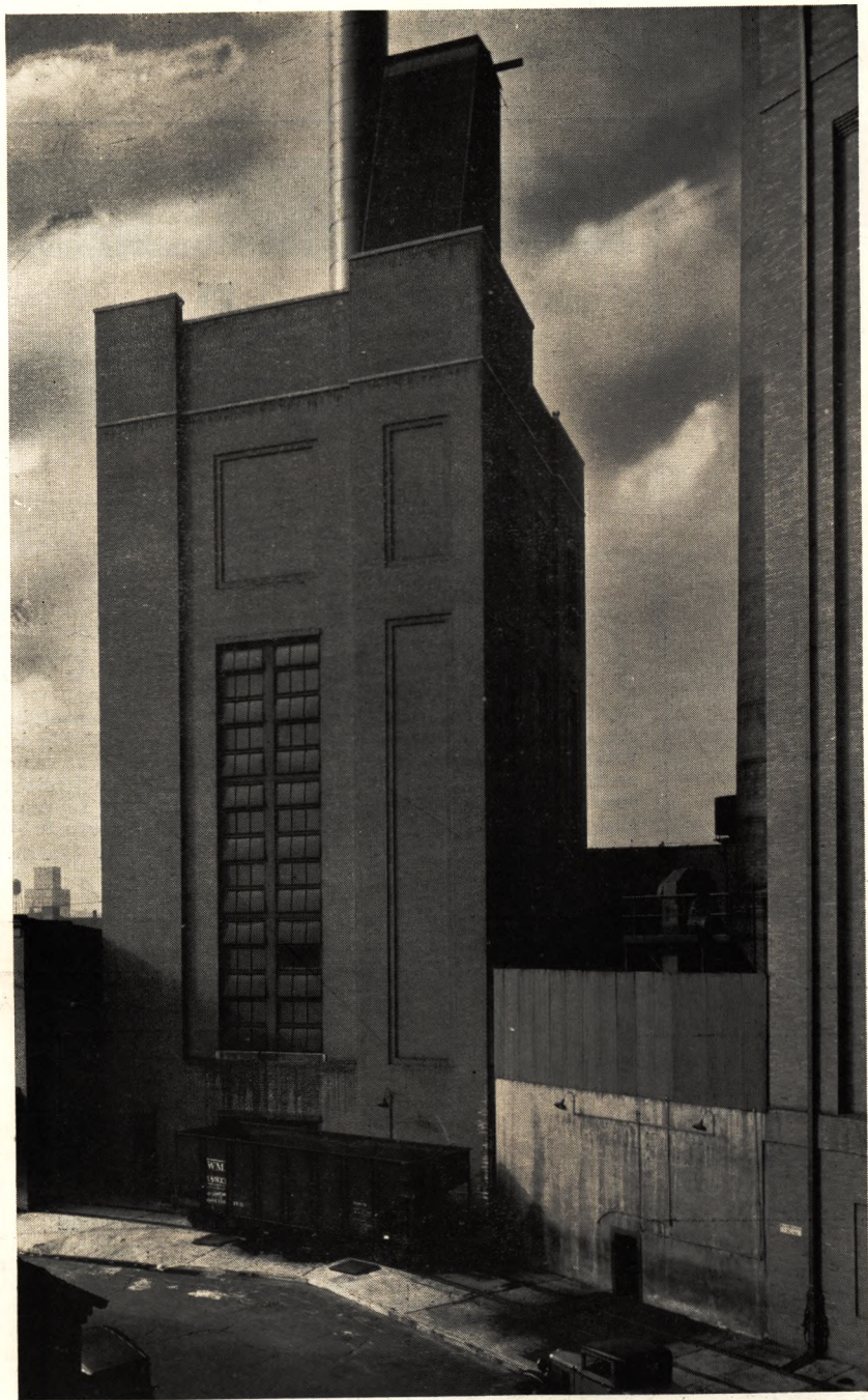
First Section of New Terminal Plant—Baltimore
