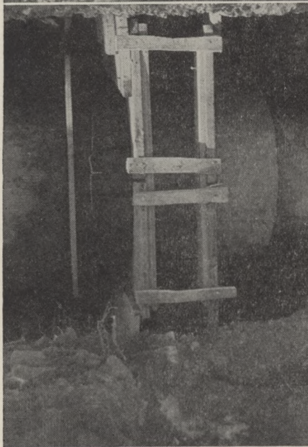
FIG. 7.—Section of Line at Expansion Joint Showing Anchor, Sheet Metal Arch, and Wooden End Forms.
