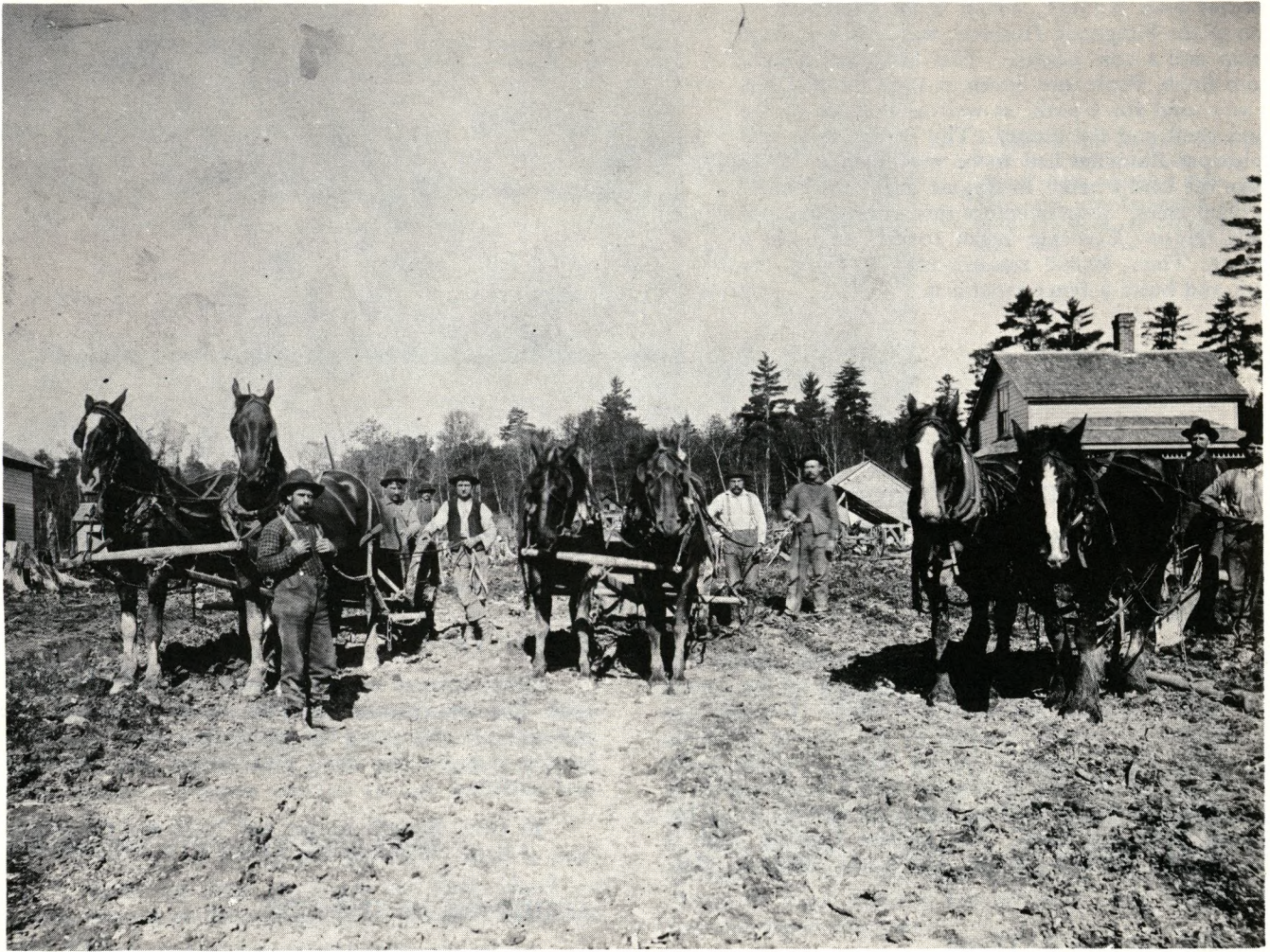
The above is a picture of the breaking of the ground for the first block of Hayes Street from Carrie Avenue to Douglas Avenue in Old Town.
