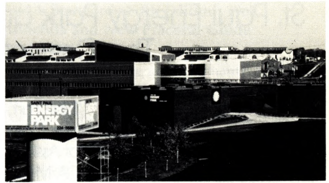
The finished plant for the St. Paul Energy Park.
