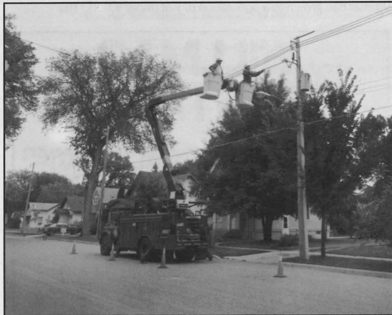
Line Department employees at work, with bucket truck
