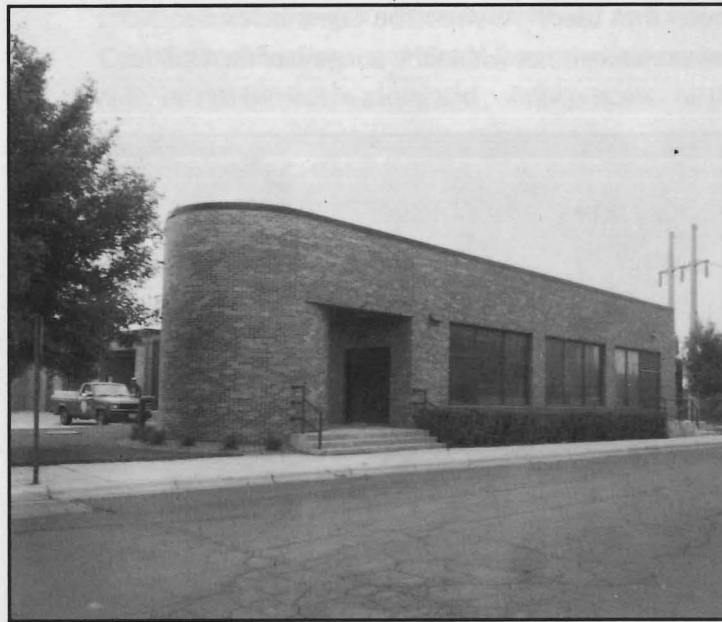
District Heating Conversion Building
