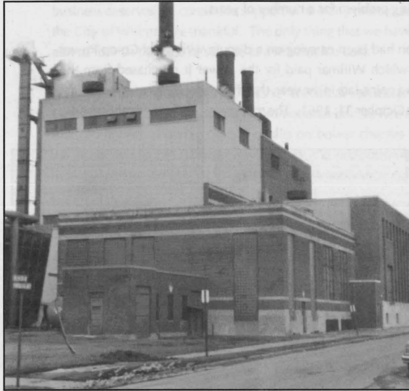
Power Plant, c. 1985
