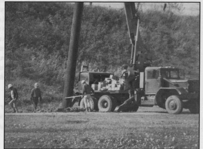
Transmission Line Construction
