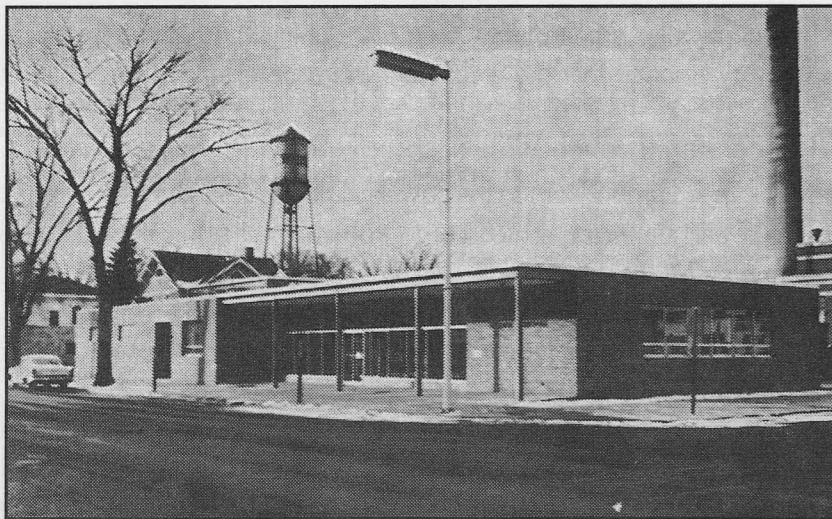
Municipal Utilities Office and Service Building c. 1957
