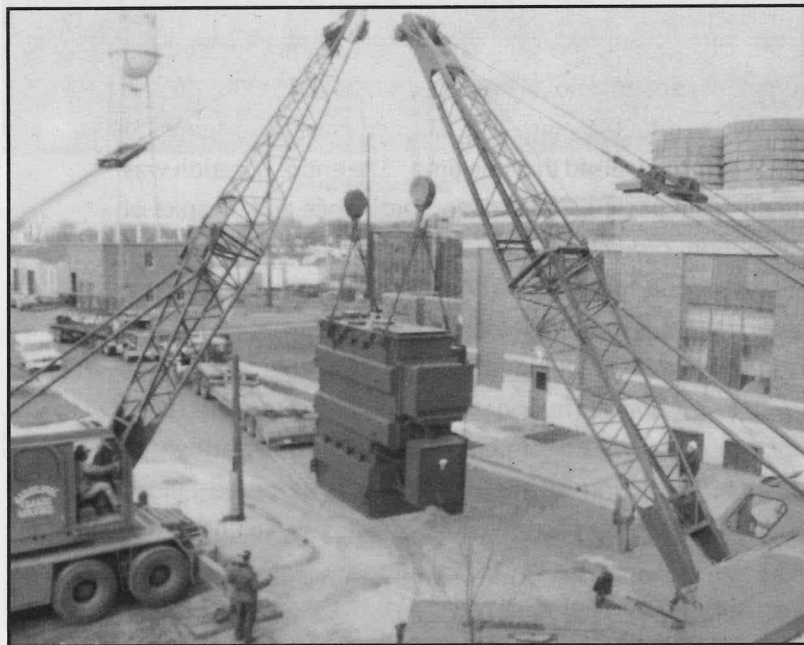
Installing power transformer near Power Plant
