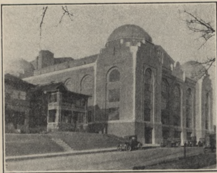
Shrine Temple, Cedar Rapids, Iowa Furnished with Steam Heat by Iowa Railway and Light Company
