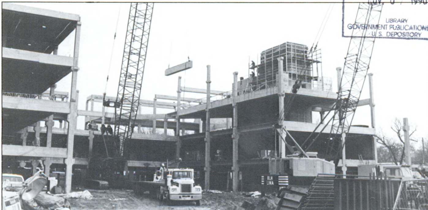
The Lancaster County Jail building, under construction in Lincoln, Nebraska, is one of two buildings targeted for district heating/cooling system operation.
