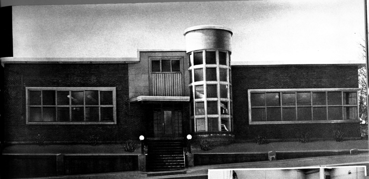
BUFFALO STREET PUMPING STATION ↑
