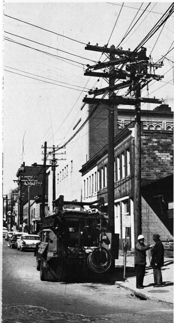
Relocating wires on new poles for street widening. Picture shows East side of Washington Street looking North from Second Street.
