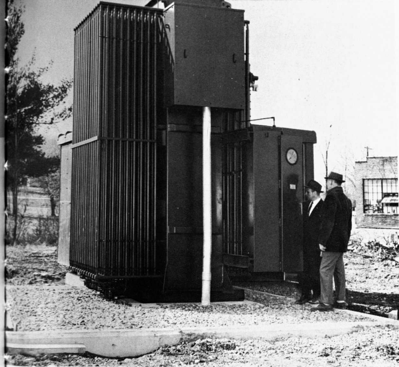
Huxley Street Substation during construction.
