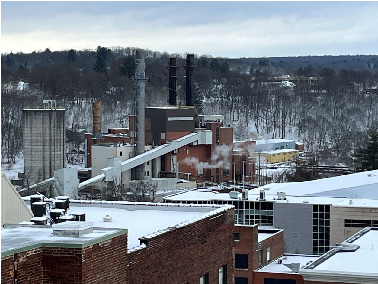
Photo 1 – Samuel A. Carlson Electric Generating Station - Photo Taken from Covenant Manor Rooftop
