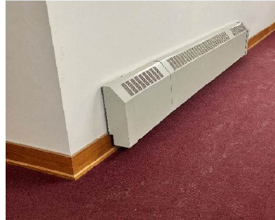
Photo 16 - Euclid Gardens - Typical Finned Tube Convector
