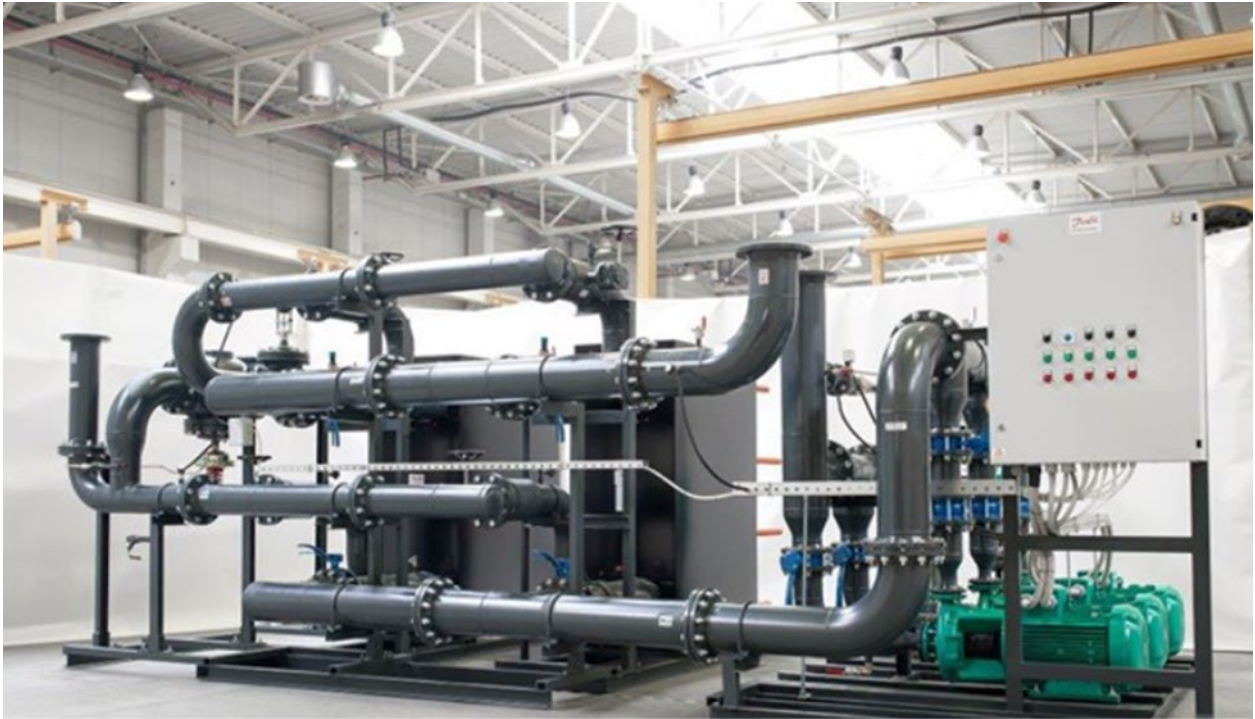
Figure 12. Typical ETS Installation (source: Danfoss)
