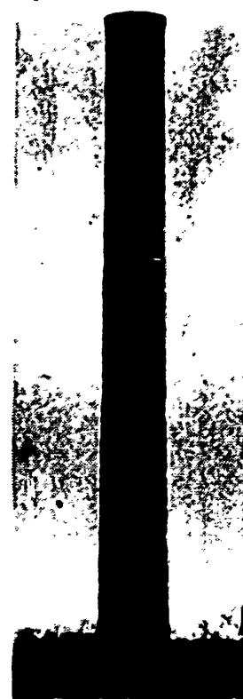
—Made Photo OLD WEST END LANDMARK Batters at Swayne Field aimed for it
