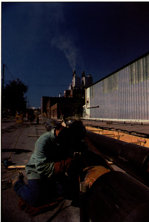
A welder connects a hot water pipe at a district heating system in Jamestown, N.Y. The system, fueled by the 25 MW cogeneration plant in the background, has 40 customers and is being expanded annually.
