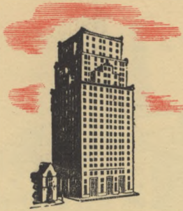
STONE & WEBSTER BUILDING 90 Broad Street, New York
