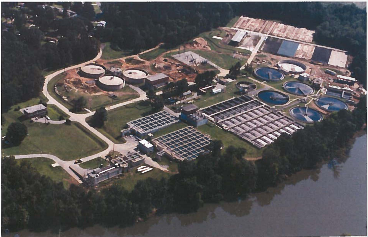
Aerial view of the South Columbus Water Resource Facility in 1990's. Construction in the background is for the new biosolids processing facility and an odor control facility.
