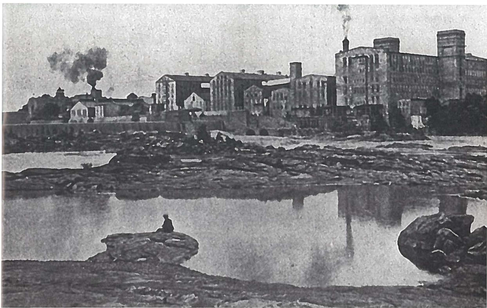
Eagle and Phenix Mill was one of several large water using textile mills making their home in Columbus, Georgia.
