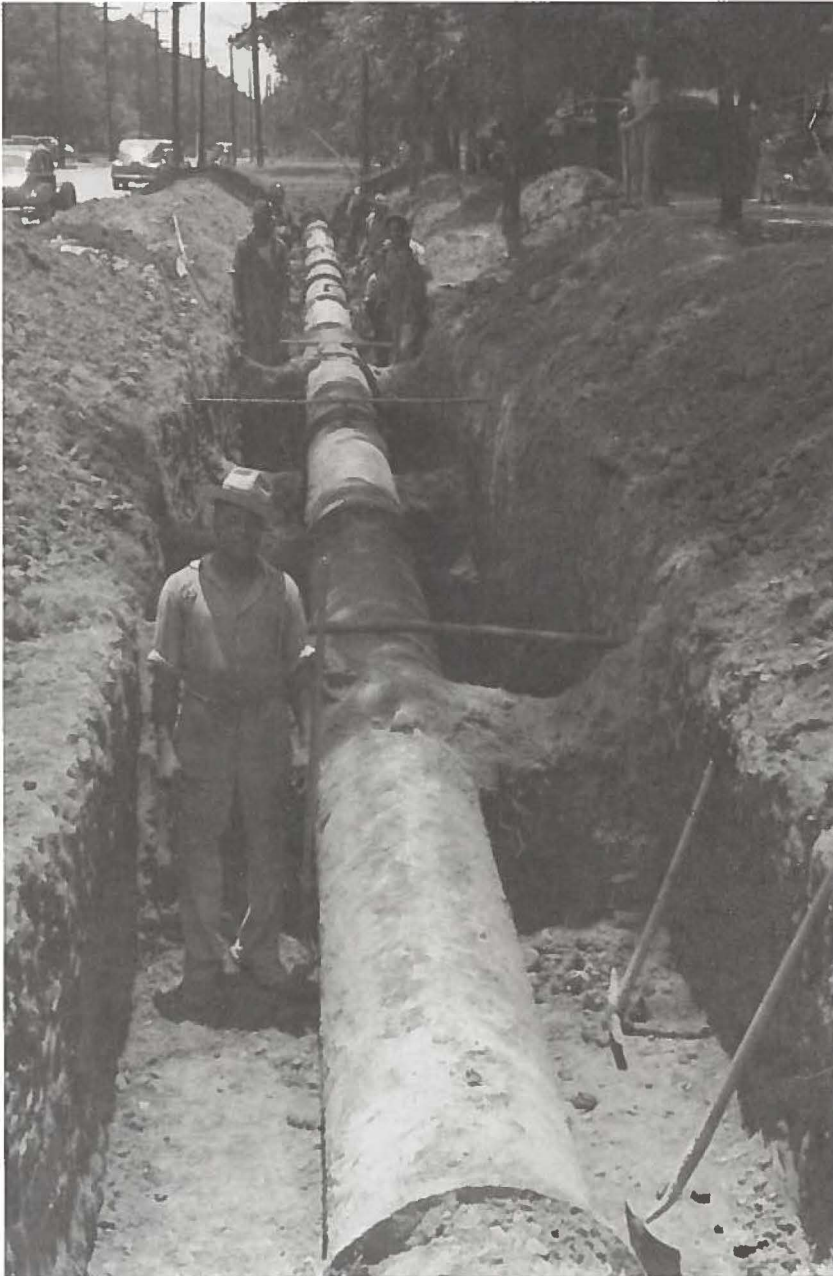
Lowering a 20-inch cast iron pipe laid in 1915 on 3rd Avenue just North of 17th Street; it's one of the main feeders from the Filter Plant into the City and is still in use today.
