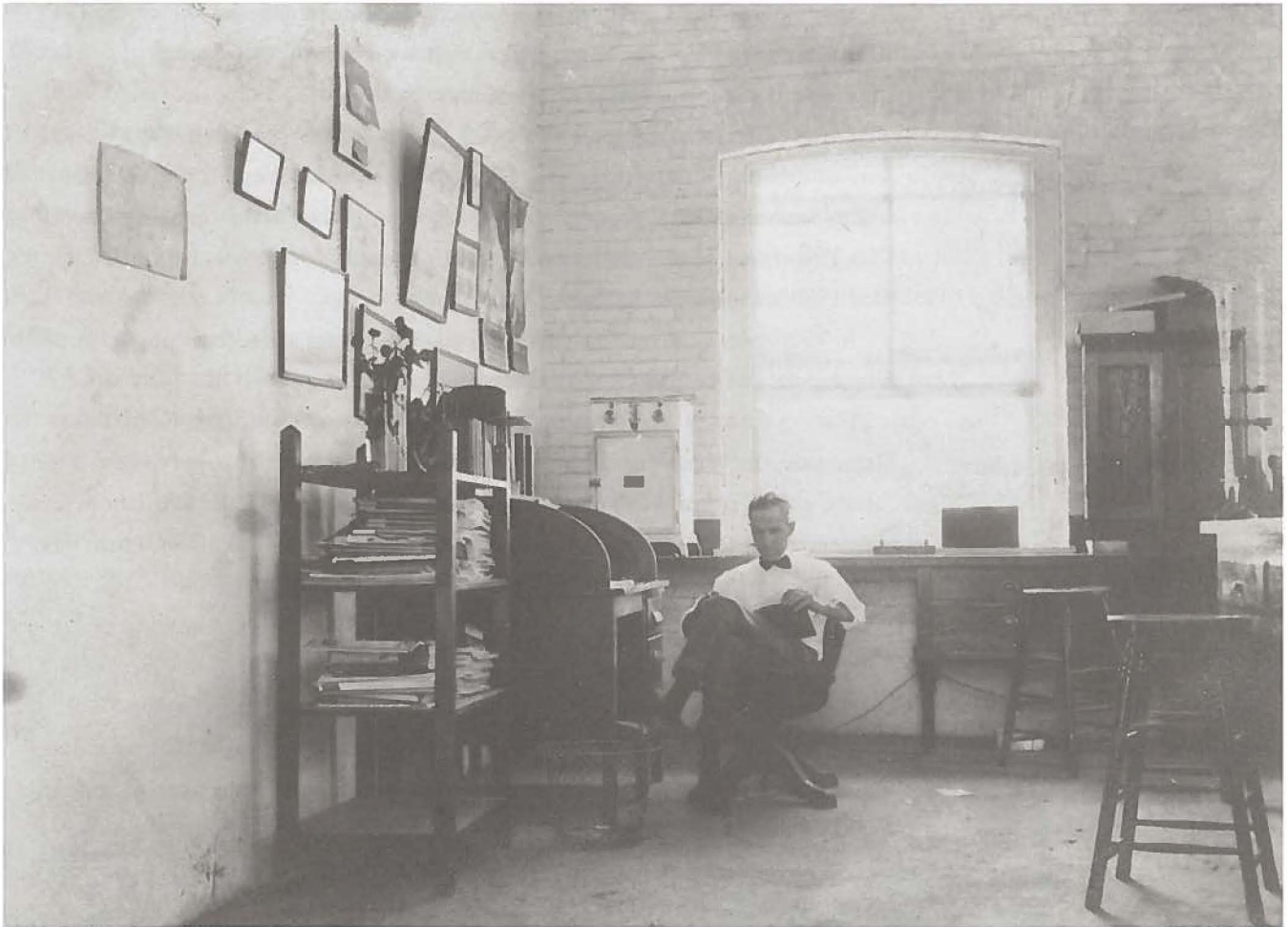
Water Treatment Plant Office and Laboratory; Dudley Chipley, Superintendent (1914-1918).
