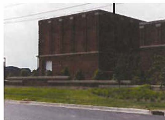
The South Commons CSO Facilities are actually located on two close but separate sites.
