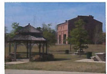
View of Uptown Park Combined Sewer Overflow Facility. The plant provides park amenities and a walking trail for public use.
