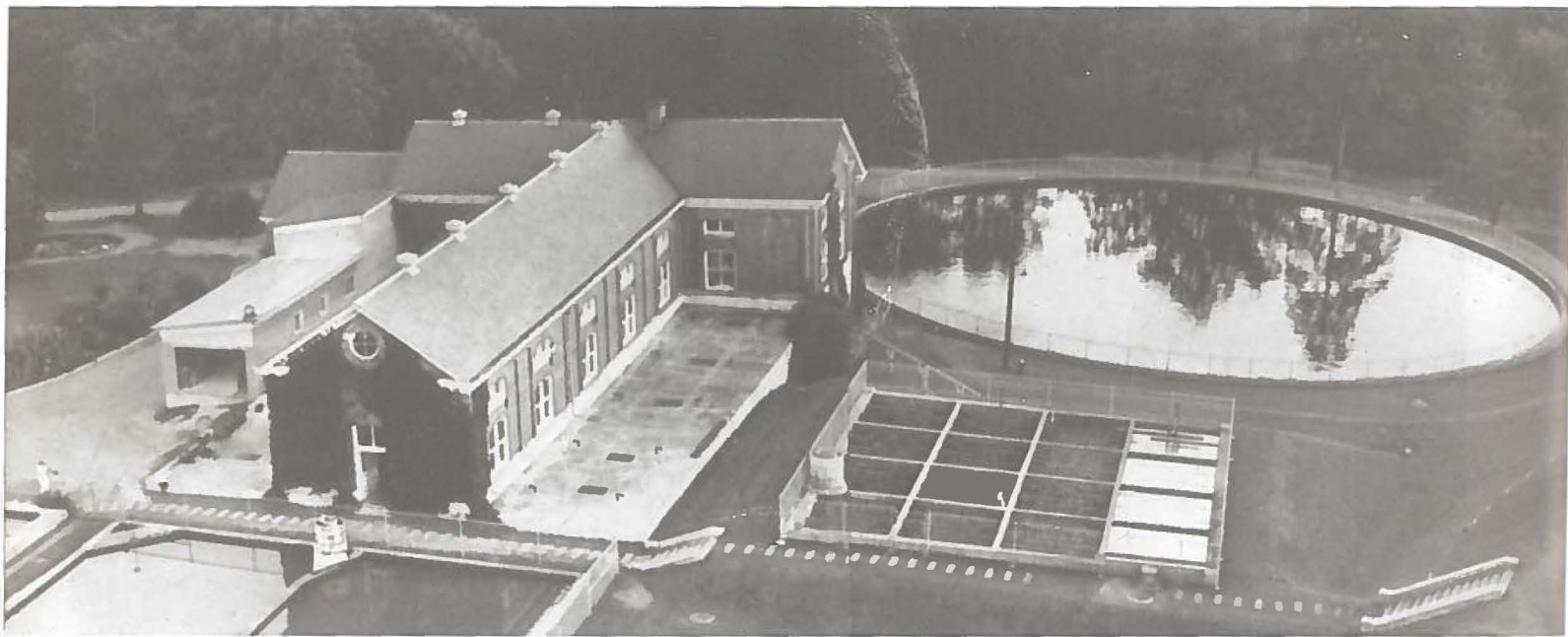
View of North Columbus Water Resource Facility water tank in 1939. Note that the finished water reservoir was open to the air. This reservoir, still in service today, was subsequently roofed over.
