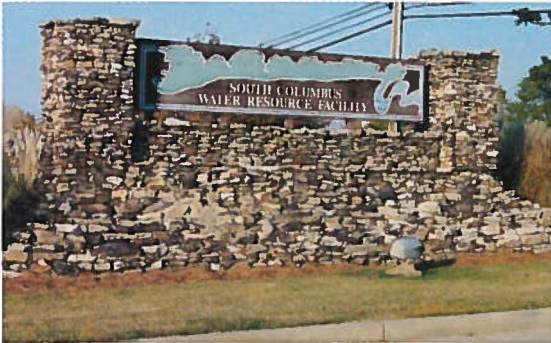
South Columbus Water Resource Facility Entrance
