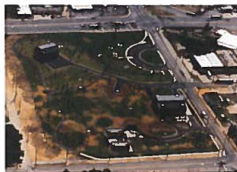
Aerial View of Uptown Park Combined Sewer Overflow Facility located between Veterans Parkway and 2nd Avenue and 18th and 19th Streets.
