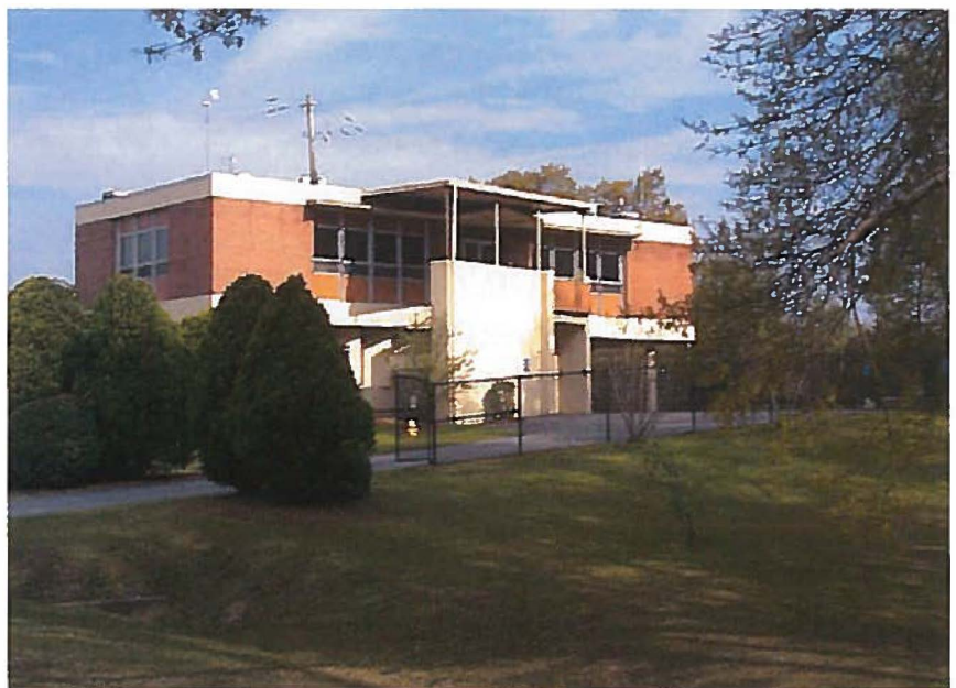
South Columbus Water Resource Facility Office
