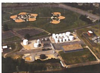
Aerial View of South Commons CSO located on Lumpkin Boulevard near the Coliseum and softball complex.
