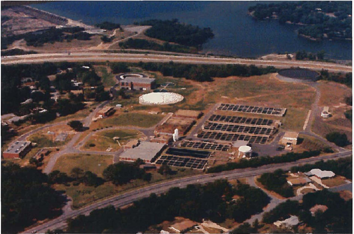
Aerial view of the North Columbus Water Resource Facility in 1990's.
