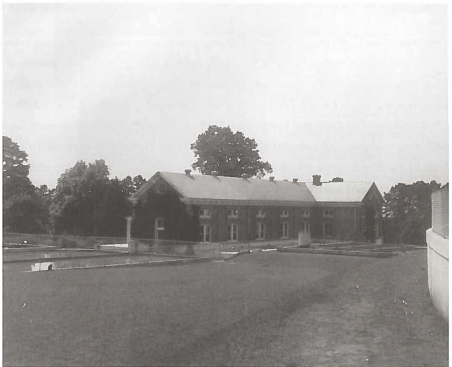
1914 – 1915 Water Treatment Plant, now called North Columbus Water Resource Facility.
