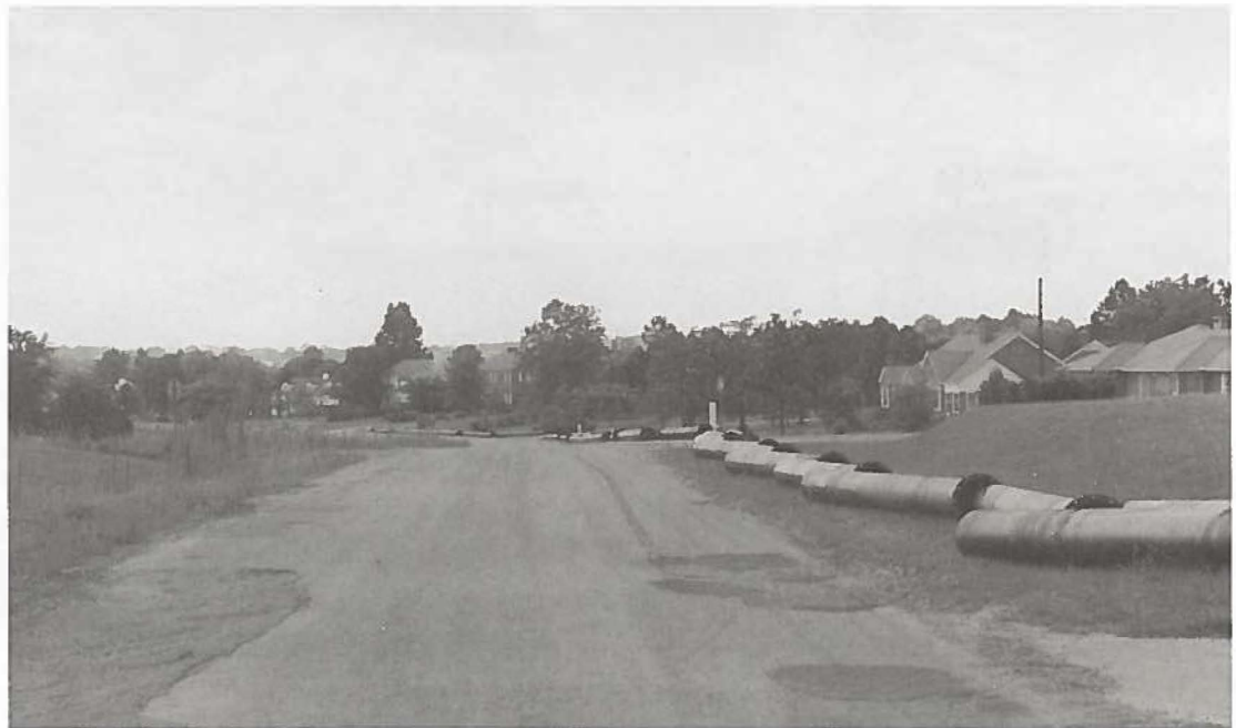
16-inch pipe ready to be installed for development on Hilton Avenue.
