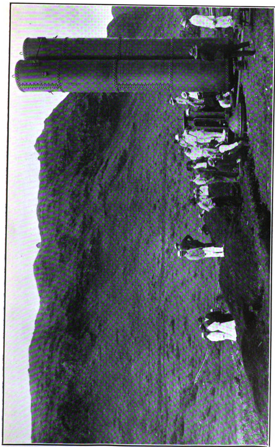
AIR CHAMBERS AT THE END OF 30" LOCK BAR PIPE LINE AT NO. 1 RESERVOIR.
