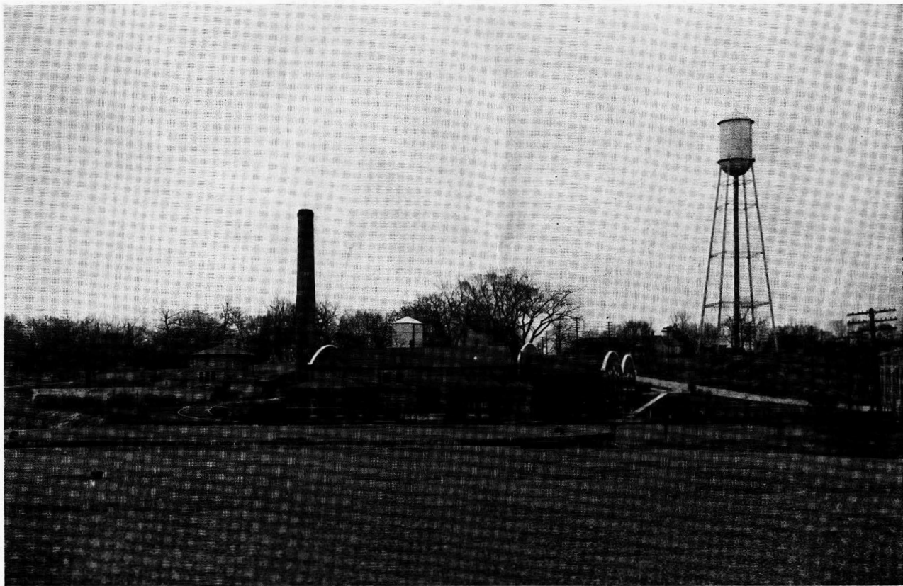
THIS IS A VIEW OF THE MAIN PUMPING STATION AS IT LOOKS AT THE PRESENT TIME. TAKEN FROM ON TOP THE STORAGE RESERVOIR.
