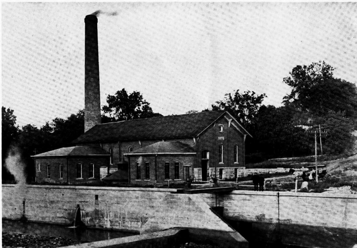
THE PUMPING STATION AS IT LOOKED BACK IN 1910. THE LARGE STRUCTURE IS THAT PART OF THE STATION BUILT IN 1876.
