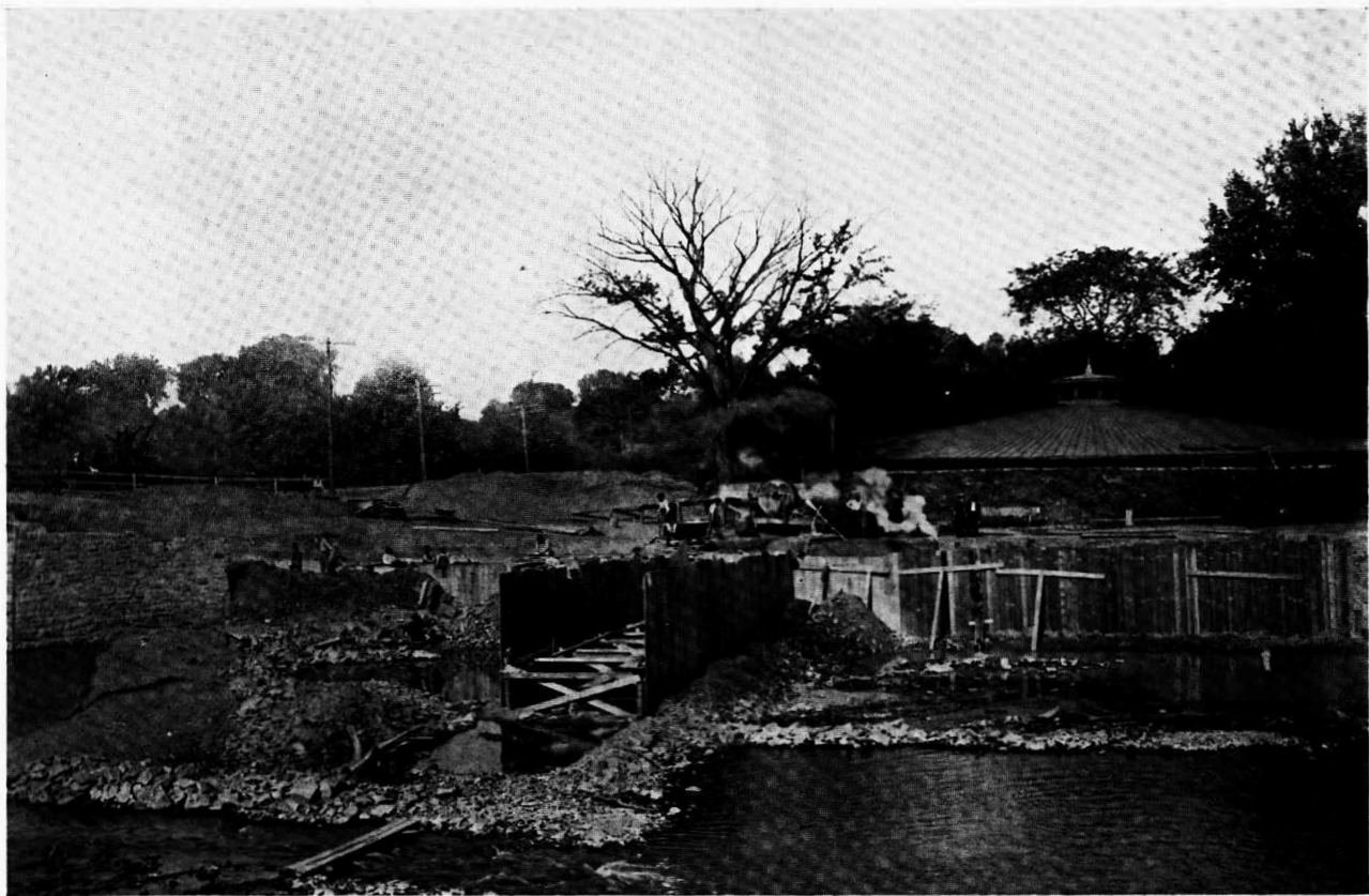
THIS PICTURE WAS TAKEN IN 1909 SOON AFTER THE ONE MILLION GALLON RESERVOIR WAS COMPLETED, WHILE THE CONCRETE DAM WAS UNDER CONSTRUCTION.
