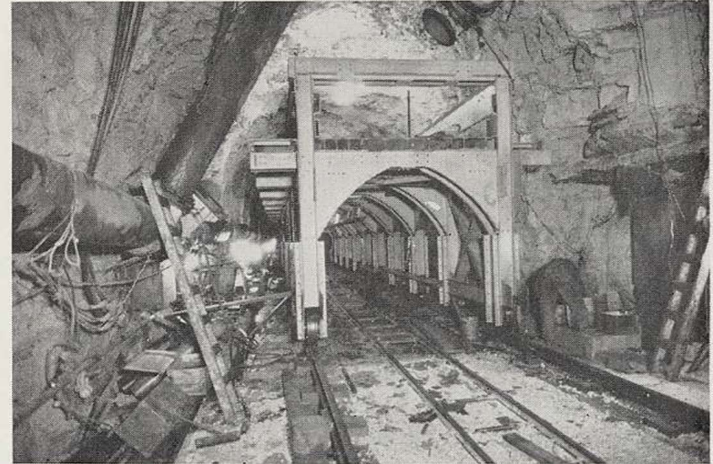
Figure 8—Rear View Mucking Machine Chicago Avenue Tunnel
