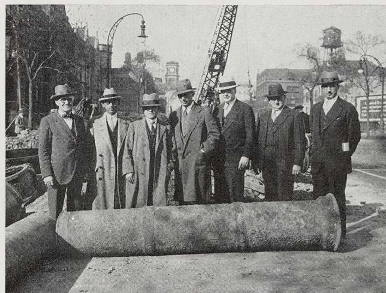
Figure 19—Section of 24-inch cast iron main laid in 1854 and removed in 1932
