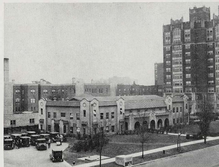
Figure 22—Experimental Filtration Plant
