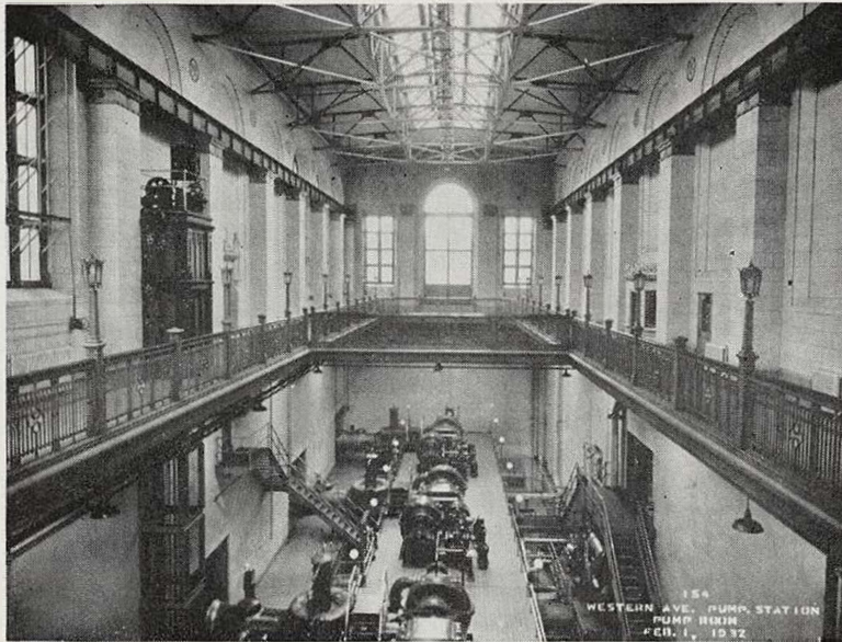
Figure 14—75 M.G.D. Turbine driven Centrifugal pumps—Western Avenue Station
