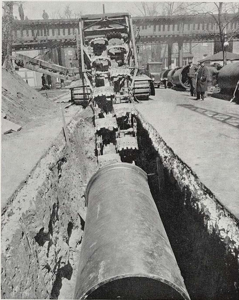
Figure 20—Laying large water main
